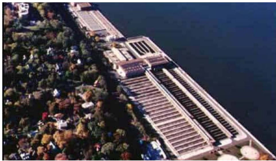
The Wastewater Treatment Plant in Yonkers, operated by Westchester County
