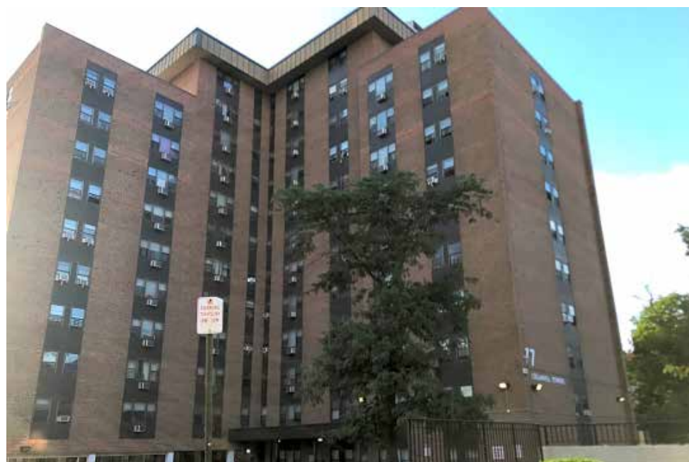
77 Locust Hill Avenue
