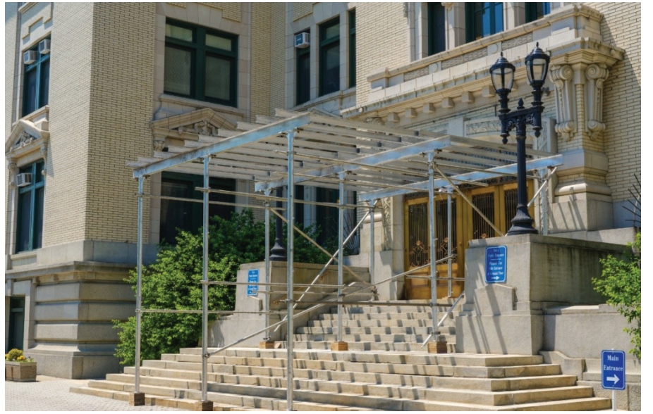
Scaffolding is being put in place this week ahead of a renovation project at Yonkers City Hall. Photo by Maurice Mercado/City of Yonkers
