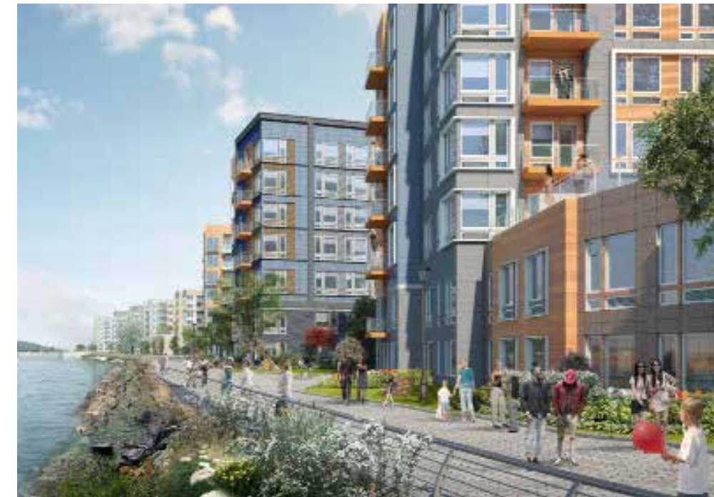
A rendering of Hudson Piers, and the public, waterfront walkways that will also be created for all
