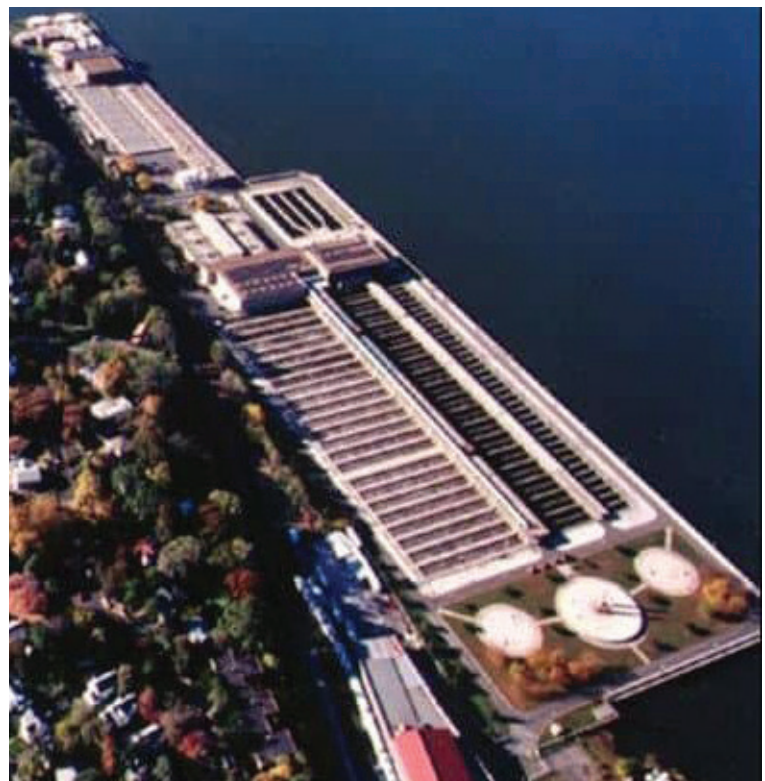
left: Yonkers Wastewater Treatment Plant
