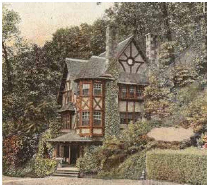
The Park Hill Train Station elevator house, part of the Getty Square Spur of the Putnam Line
