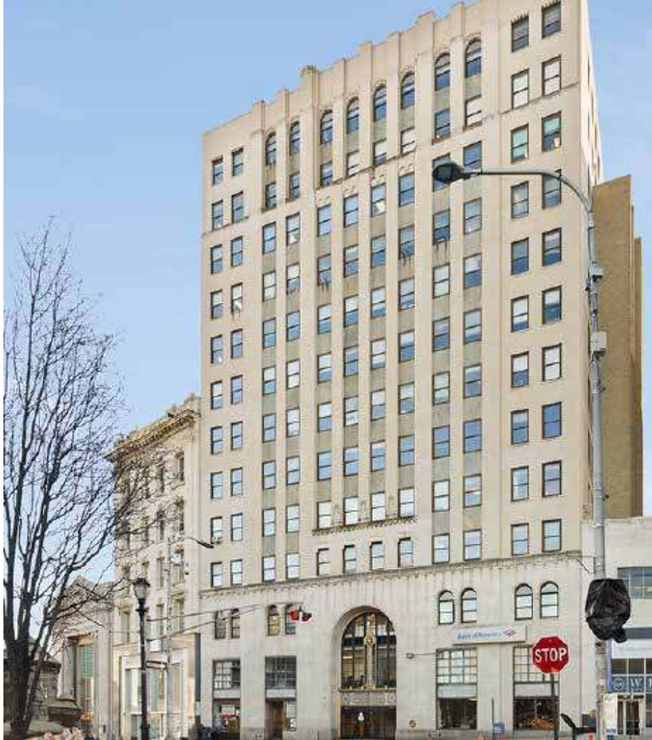
County Department of Health Office, 20 South Broadway
