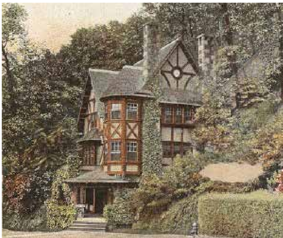
Lower elevator house for the Park Hill elevator
