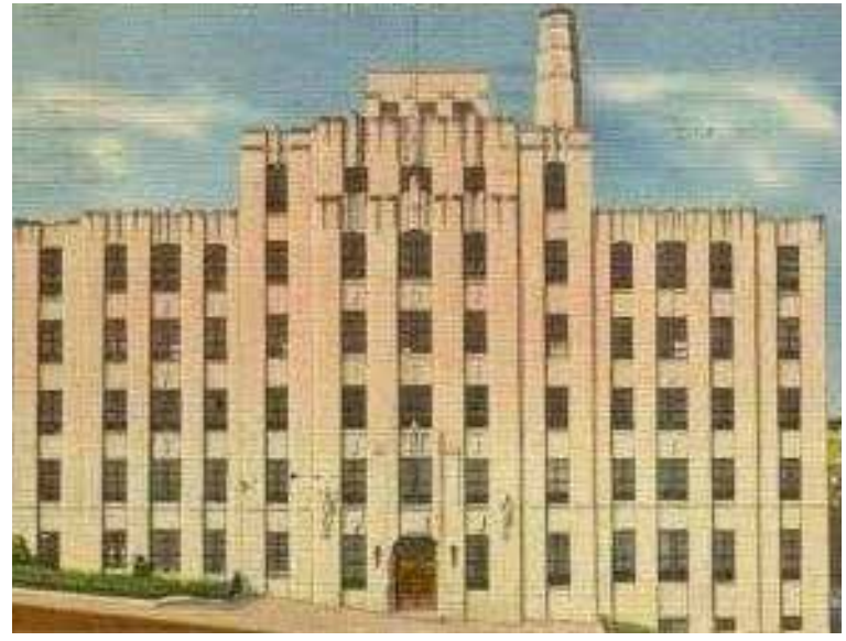
The Yonkers Health Center, one of the first comprehensive full service municipal clinic and research facilities in the country. Now it is used for City of Yonkes offices
