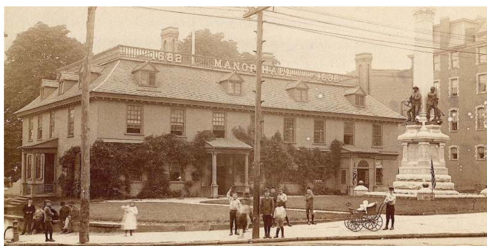
Philipse Manor Hall, the oldest building in Yonkers
