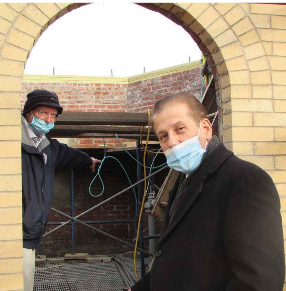
City Councilman Anthony Merante, right, with City Engineer Paul Summerfeld, in the water tower at Sprain Lake.
