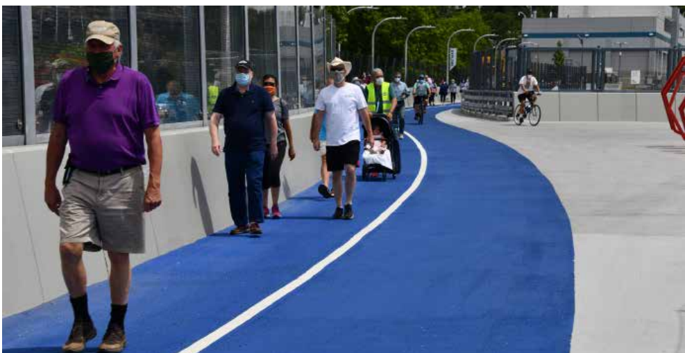
walkers enjoy the new walkway path on the Mario Cuomo Bridge
