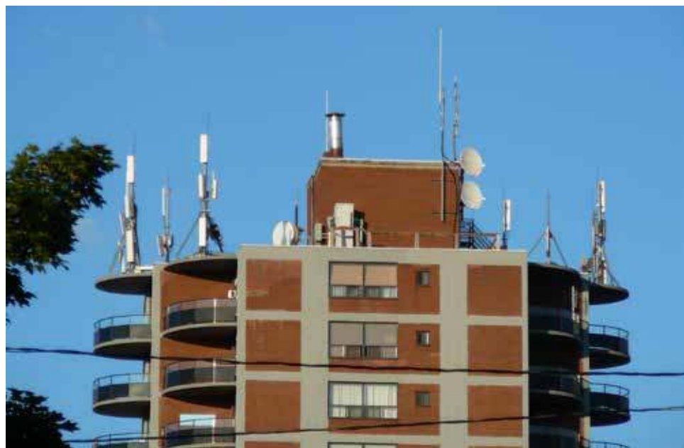
Many Westchester apartments and co-ops have permitted cell phone towers on their roofs for additional income
