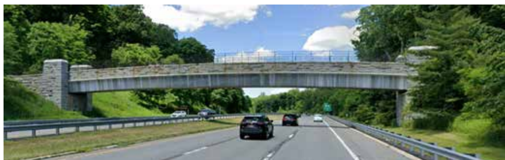
Taconic Parkway pedestrian bridge from Google Maps
