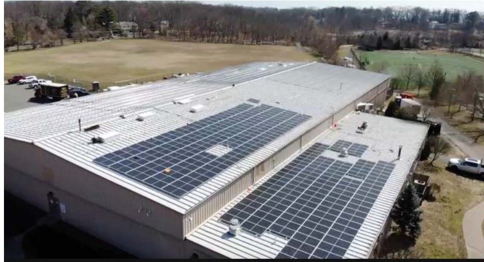
Solar panels at the Town of Mamaronecks Hommocks Park Ice Rink
